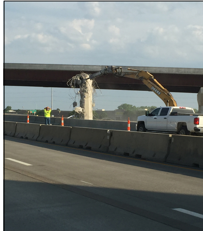
The pier shown above was removed last weekend at the I-35/K-435 interchange, as seen at right.
