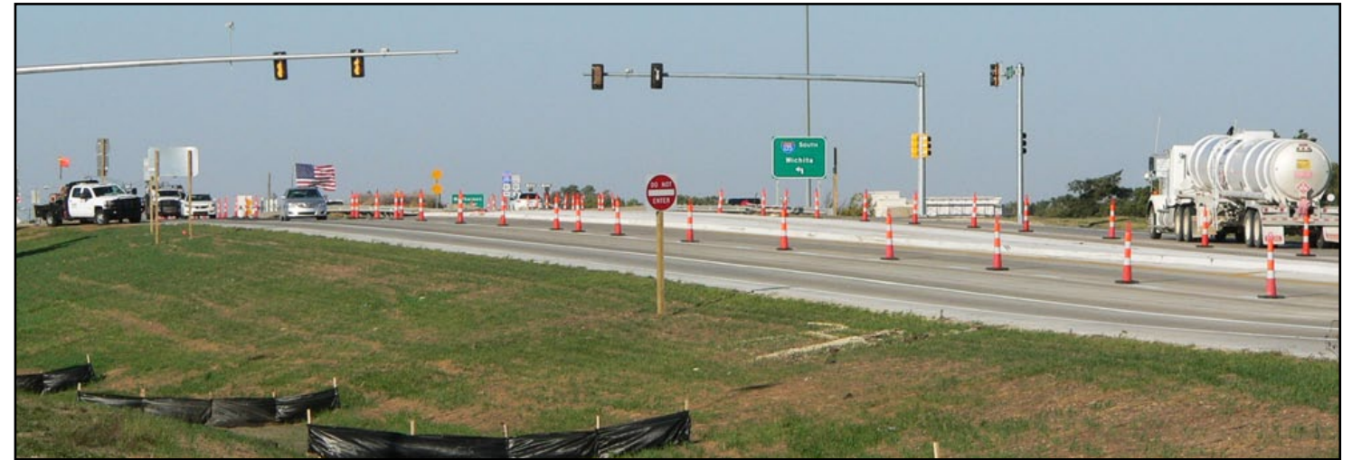
Improvements are finishing up at the U.S. 56/I-135 interchange in McPherson.
