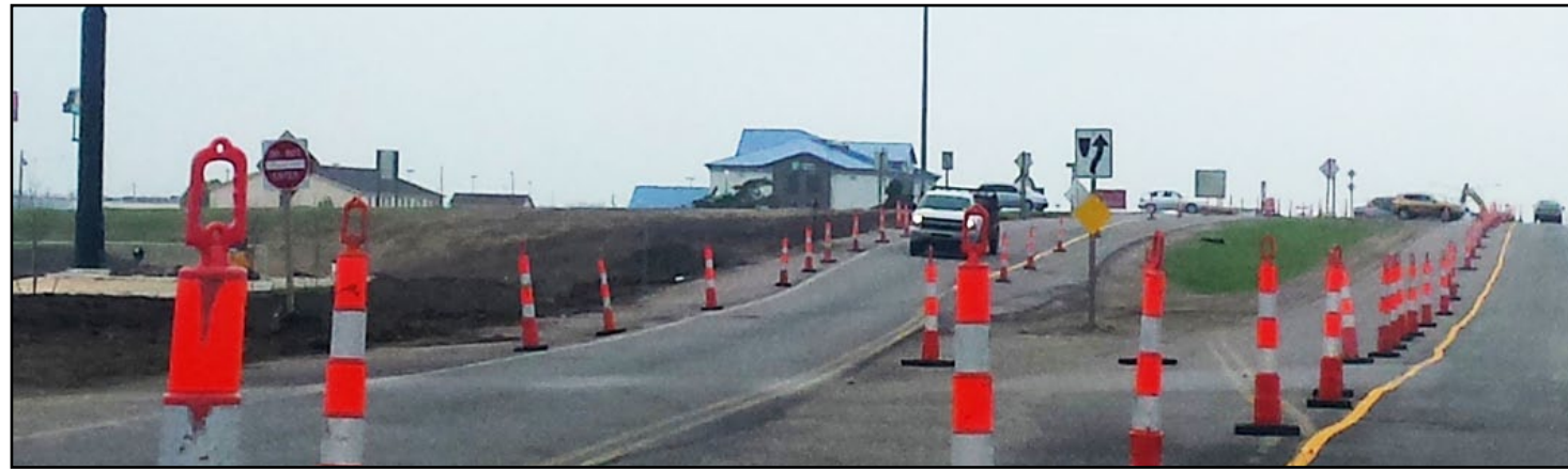
Construction improvements to U.S. 56 near McPherson should be completed this fall.
