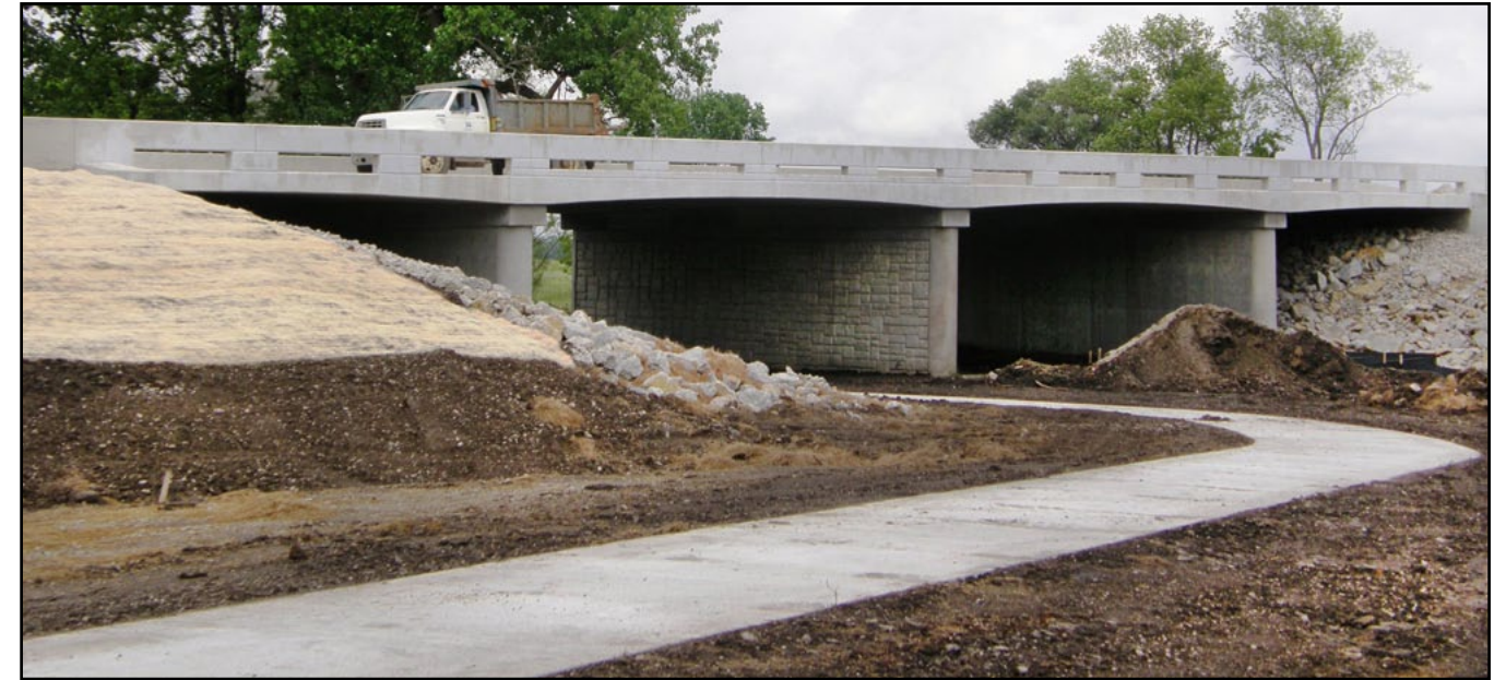
At left is the old railroad overpass on K-39 at the eastern edge of Chanute, and below is the new bridge that has replaced it. B&B Bridge of St. Paul was contractor on the $1.7 million project, which lasted one year. The new bridge has a 44-foot roadway and is lower than the previous structure. A section of the Katy Hike/Bike Trail that runs underneath was paved as part of the project.
