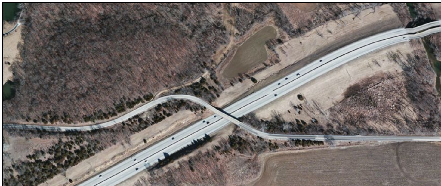
Reconstruction of the Kansas Avenue Bridge in Leavenworth County crossing over the KTA/I-70 near mile marker 221 is set to begin soon. The bridge has deteriorated to the point it needs to be replaced and was closed to all traffic last week. AM Cohron & Sons is the contractor for the project that should be completed in November. Most bridges crossing the KTA are 50 years or older.
