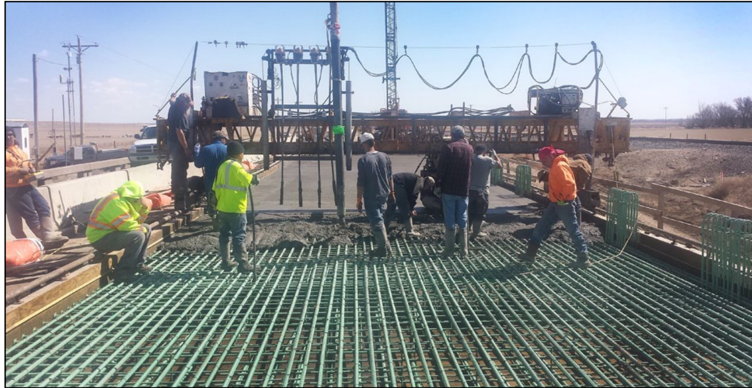
Contractors place concrete on the U.S. 50 bridge deck earlier this month.
