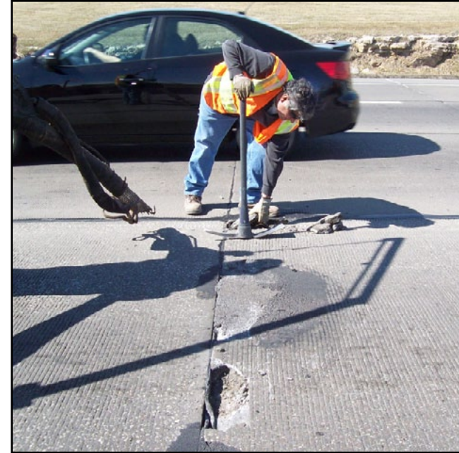
Pothole season is in full swing in the Kansas City Metro area. At left, Equipment Operator Ruben Hernandez from the Lamar Subarea Office spray patches a pothole on I-35 just north of the Lamar shop. Above, another pothole nearby gets repaired.
