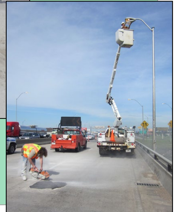
Multitasking is the name of the game when maintenance crews close down two of three lanes on U.S. 54 in west Wichita. The West Wichita Subarea crew patched bridge potholes (above) while the lighting contractor took advantage of the traffic control and changed out light bulbs (right). The Average Annual Daily Traffic (AADT) count on this section of U.S. 54, just west of I-235, is 87,800.
