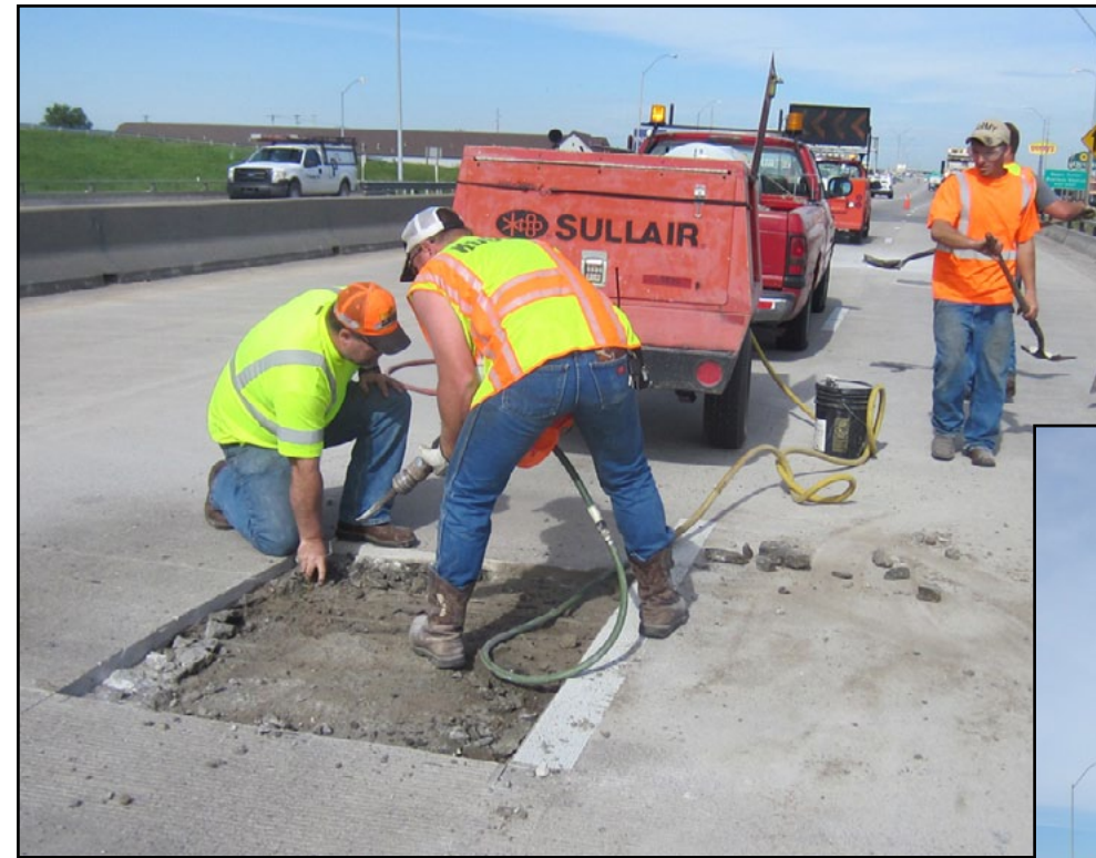
Multitasking is the name of the game when maintenance crews close down two of three lanes on U.S. 54 in west Wichita. The West Wichita Subarea crew patched bridge potholes (above) while the lighting contractor took advantage of the traffic control and changed out light bulbs (right). The Average Annual Daily Traffic (AADT) count on this section of U.S. 54, just west of I-235, is 87,800.
