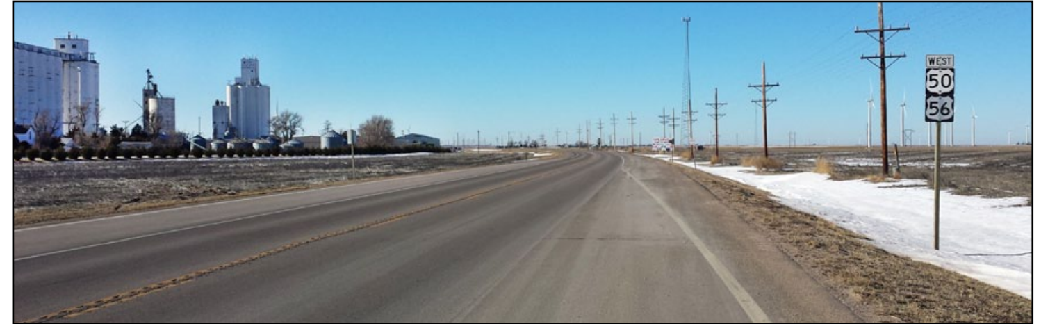
A preliminary engineering study is taking place on this section of U.S. 50.
