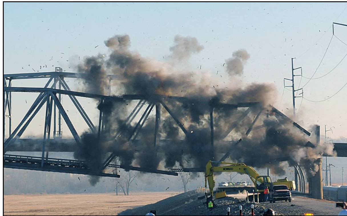
The first section of the U.S. 69 bridge is imploded.
