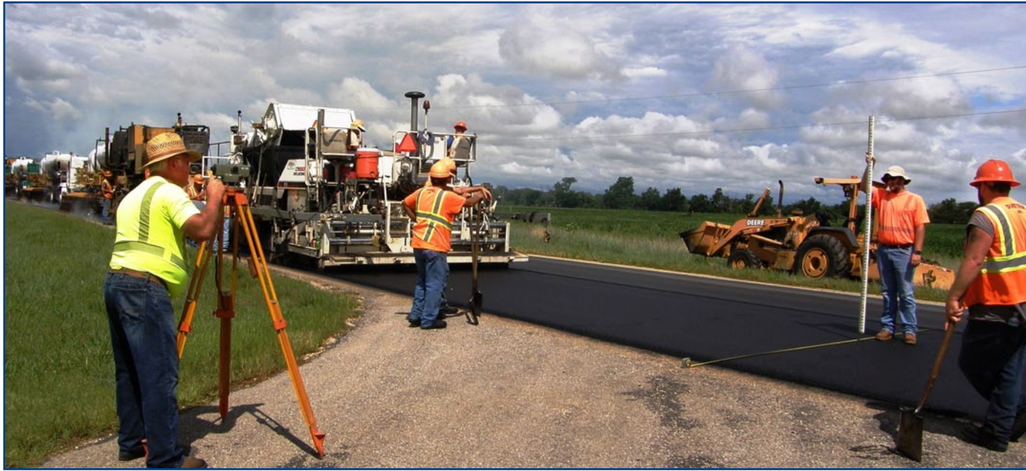
KDOT inspectors Wade Park, left, and Warren Ebberts of the Iola office measure the surface recycle on a recent preservation project on K-58 between Leroy and U.S. 75. The surface recycle was followed by a chip seal. Dustrol, Inc., of Towanda was awarded the $285,801 construction contract.
