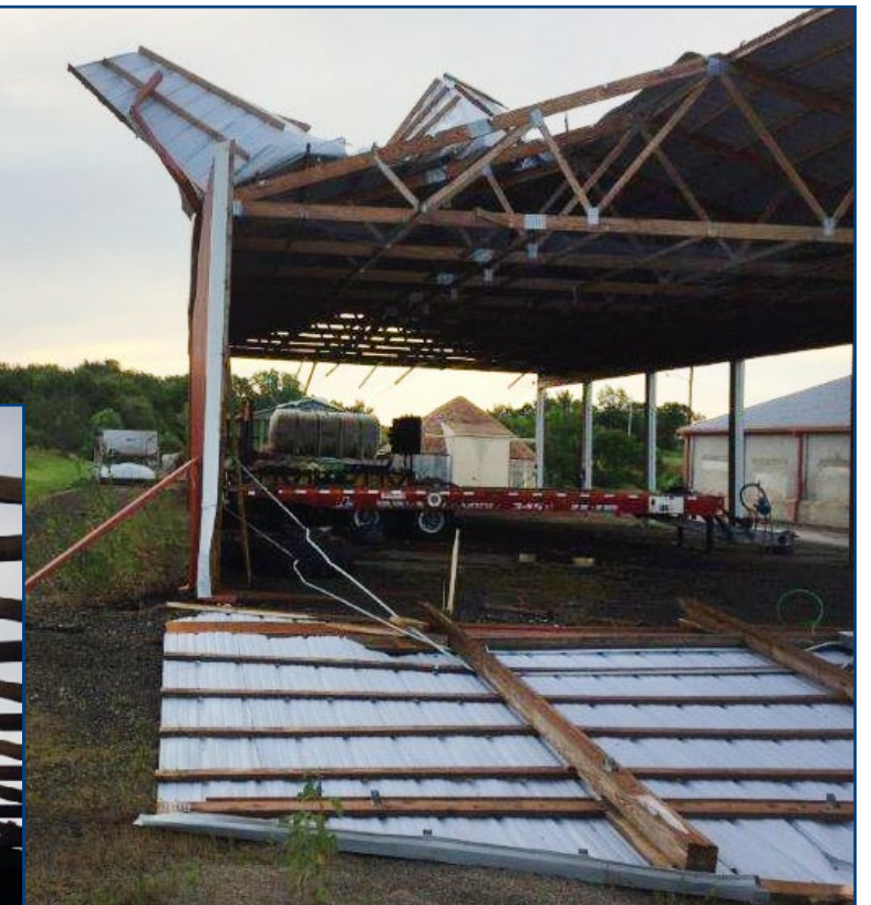
The storm damage includes destruction of the equipment shed (above), roof blown off the sand/salt materials shed (left) and several broken windows in the Subarea shop.
