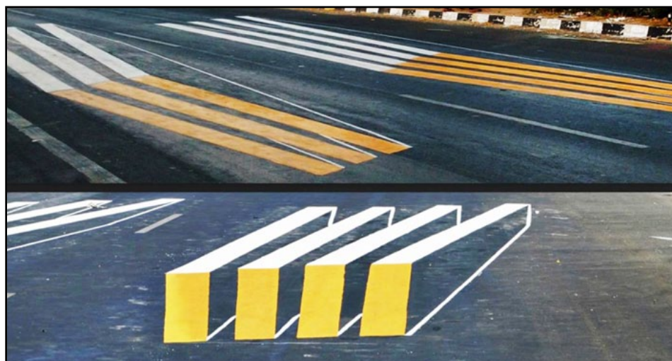
The crosswalk design is painted as a stretched out chevron design and appears as such when viewed from the side.
