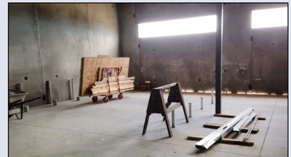
Renovations continue at the Matfield Green service area.
