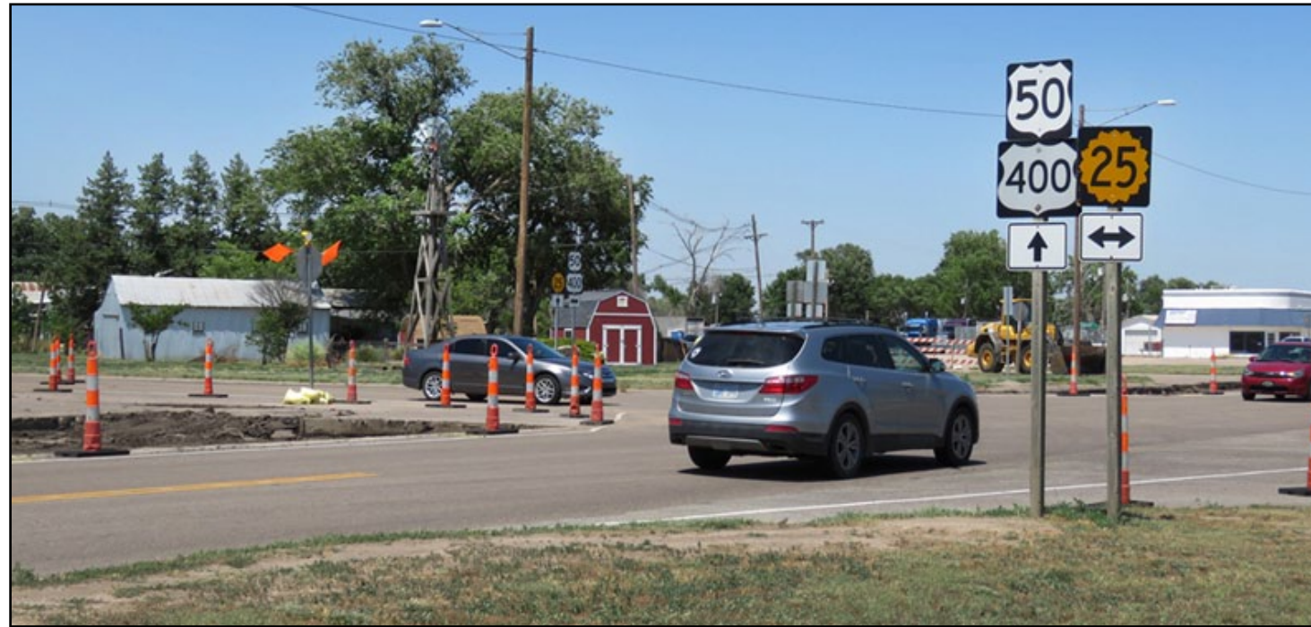
Improvements have begun at the U.S. 50/K-25 intersection in Lakin.
