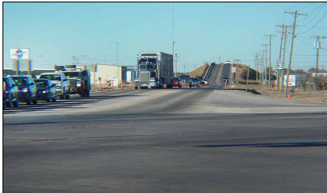
Construction continues on the U.S. 54/U.S. 83 intersection in Liberal.
