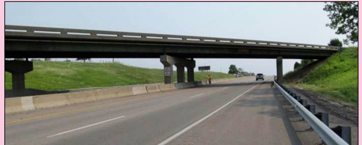
Replacement of the K-32 bridge over I-70/KTA is underway.
