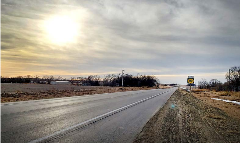
Above, the new highway features a wider driving surface as well as 6-foot paved shoulders. At right, new pavement and profile on K-383 near Woodston. The hills in this area were cut down to help improve motorist visibility. Photos by Lisa Mussman, District Three
