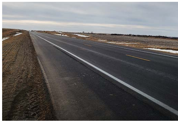
Above, the new highway features a wider driving surface as well as 6-foot paved shoulders. At right, new pavement and profile on K-383 near Woodston. The hills in this area were cut down to help improve motorist visibility. Photos by Lisa Mussman, District Three
