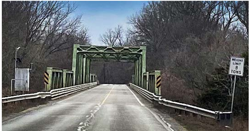
Two of the bridges that will be replaced under the revamped local bridge improvement programs are the Neosho River bridge on old 169 highway north of Chanute (above) and the bridge over Pumpkin Creek on Montgomery County Road 1800 (old 166 highway) east of Coffeyville (below). Photos by Priscilla Petersen, District Four
