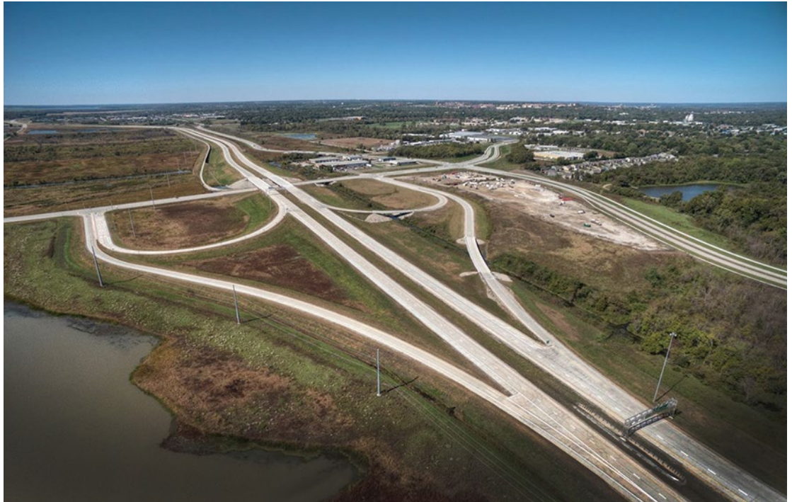
Work on the South Lawrence Trafficway, like the Haskell Avenue Interchange seen above, has been taking place for nearly 40 years. Projects on the final northern portions of the SLT were moved into the IKE Construction Pipeline in September. File photo
