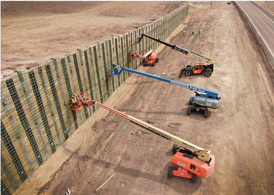
Above, a retaining wall is being constructed as part of the four-lane expansion project on U.S. 50 in Ford County. The wall is needed to preserve the historical “Point of Rocks” location near the westbound lanes. Thomas Husa’s road squad and Brad Rognlie’s bridge squad designed the project. Below, new concrete is placed for U.S. 54 expansion in Seward County. Steve Rockers’ road squad and Peter Tobaben’s bridge squad designed the project. Photos by Tim Nichols, District Six
