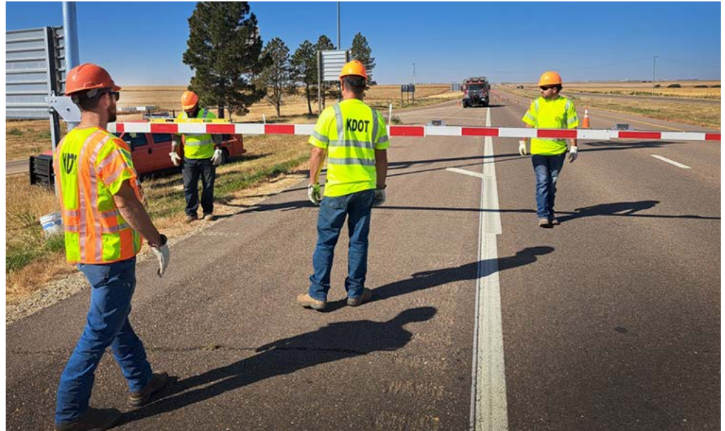
Crew members install and test out the new drop-arm snow gate on eastbound I-70 near Colby. Photos by Kenny Stewart, District Three
