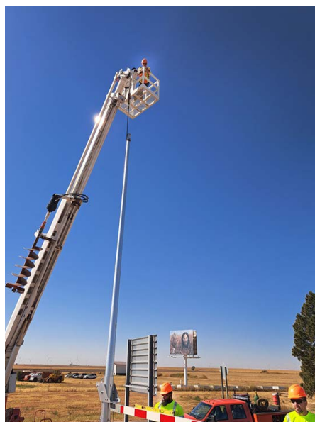
Crew members install and test out the new drop-arm snow gate on eastbound I-70 near Colby. Photos by Kenny Stewart, District Three
