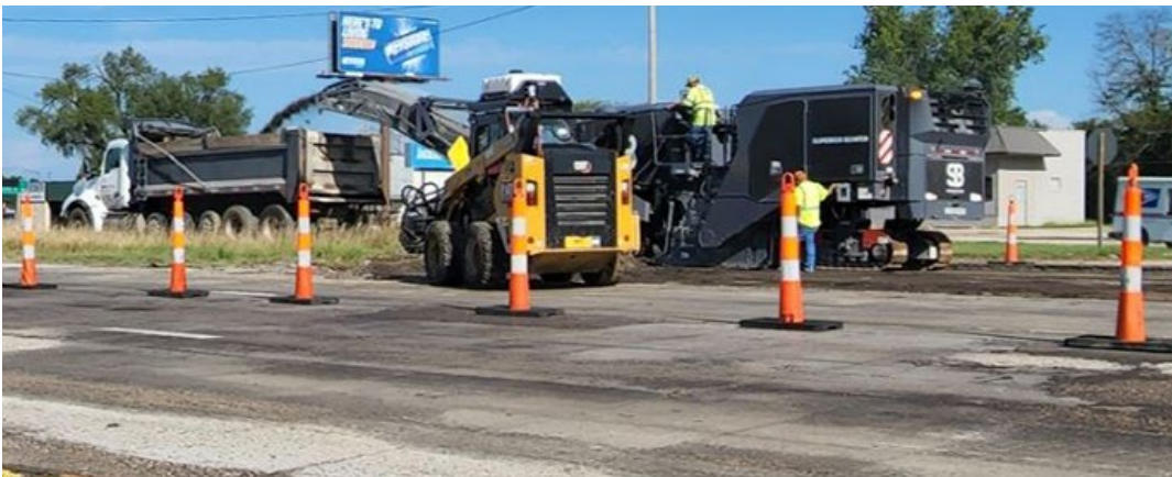
Top photo, bridge repairs on K-4 reduce traffic to one lane controlled by a signal. Above, A routine bridge inspection is done on the southbound U.S. 75 overpass. At left, milling is done on U.S. 24 near the Rochester Road intersection. Photos by Kate Craft, District One, and KDOT Multimedia Services
