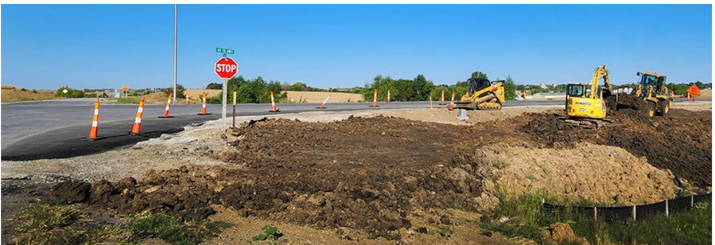
Crews working at the U.S. 75/260th Street intersection.
