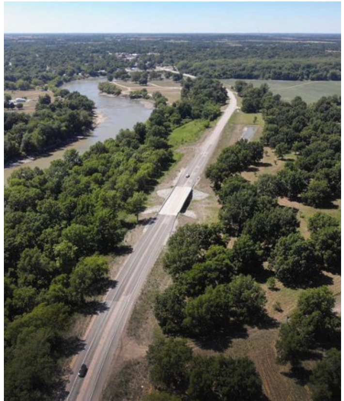
Drone footage captures one of the newly finished bridges on U.S. 166 east of Chetopa. Photo by Andrew Wilson, District Five
