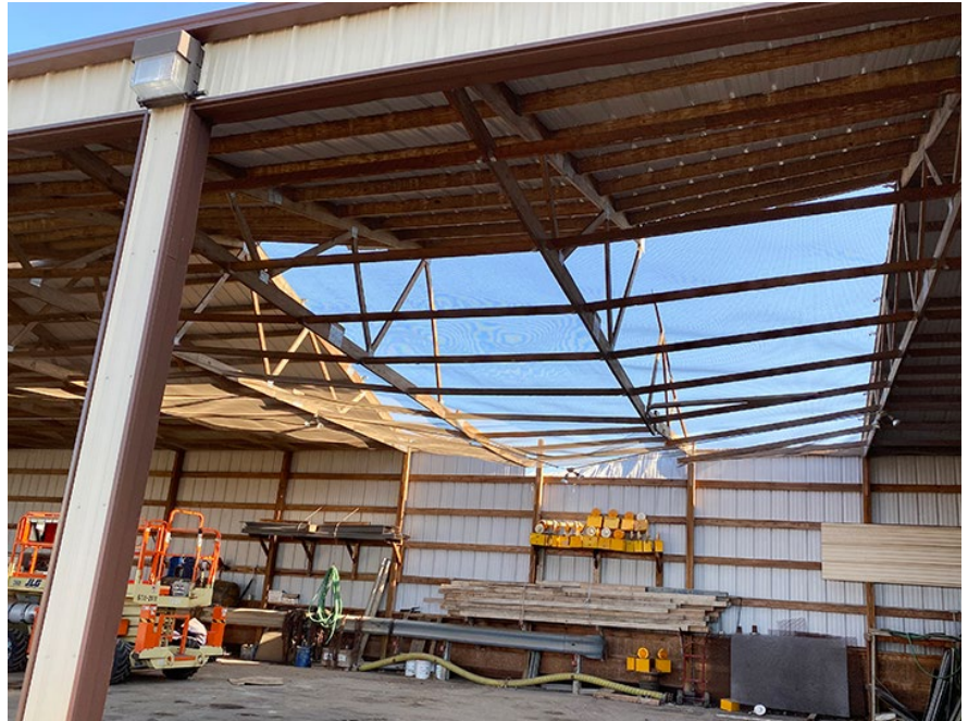
Aftermath of damage to the equipment shed at the Ellsworth Subarea following high winds after midnight on April 23.
