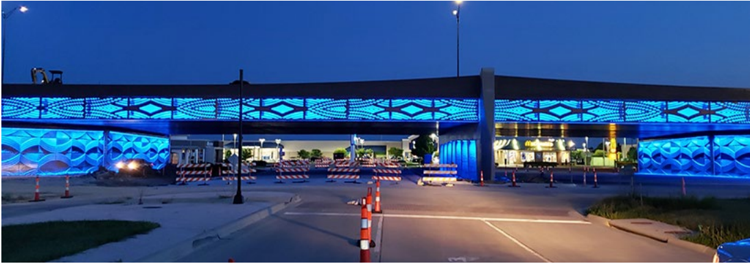
Bridge lighting is a feature on the U.S. 54 portion that received awards.
