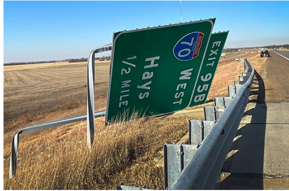
At left, signs across central and western Kansas, like the one below, were damaged in high winds on Dec. 15. Below, burned ground lines both sides of U.S. 281 in northern Russell County.
