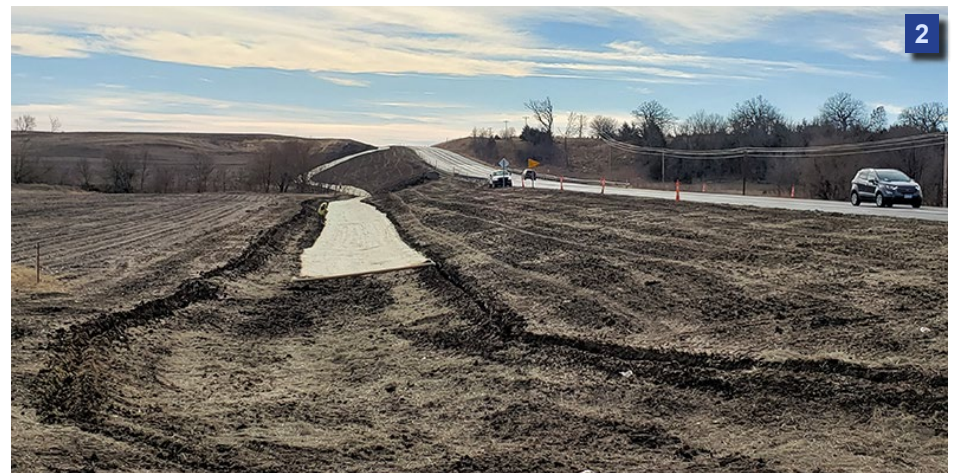
1. Contractors work on the U.S. 75 southbound passing lane in Brown County. 2. Erosion control is placed on Brown County project. 3. Contractors work on northbound portion in Jackson County. Photos by Kate Craft, District One
