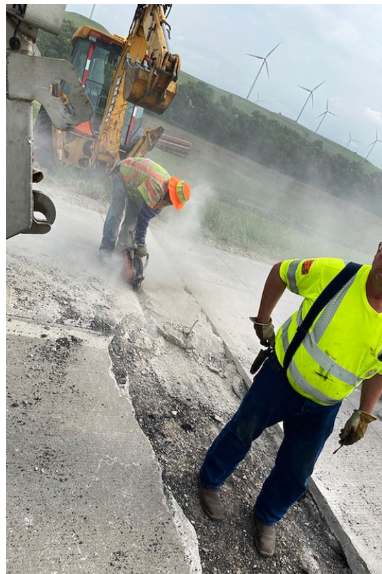
Top left, I-70 pavement in Ellsworth County buckled recently. Above, the Ellsworth Area crew responded and removed the damaged section of roadway. Below, I-70 is repaired and open to traffic. Photos by Tim Hays, District Two
