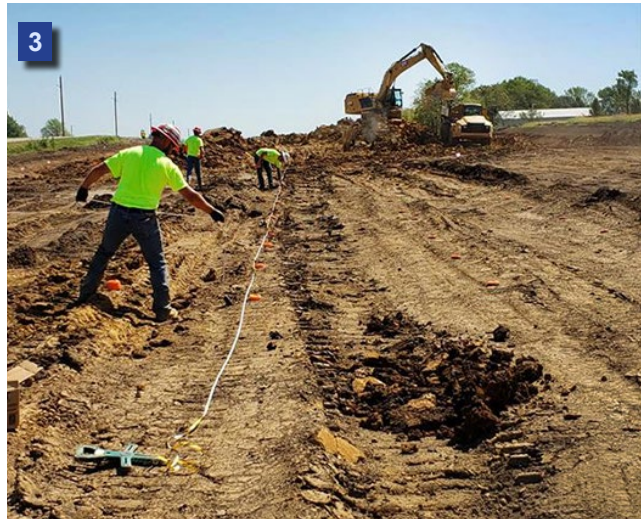
1. Blaster-in-charge checks the area before giving the all clear. 2. Equipment moves material from the post blast excavated area. 3. Workers measure tomorrow's blast grid. Photos by Kate Craft, District One
