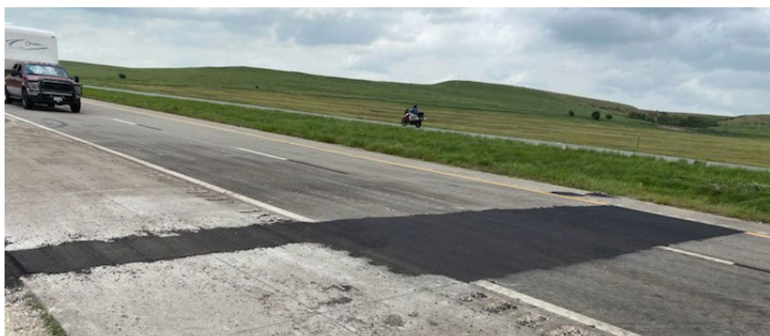
Top left, I-70 pavement in Ellsworth County buckled recently. Above, the Ellsworth Area crew responded and removed the damaged section of roadway. Below, I-70 is repaired and open to traffic. Photos by Tim Hays, District Two
