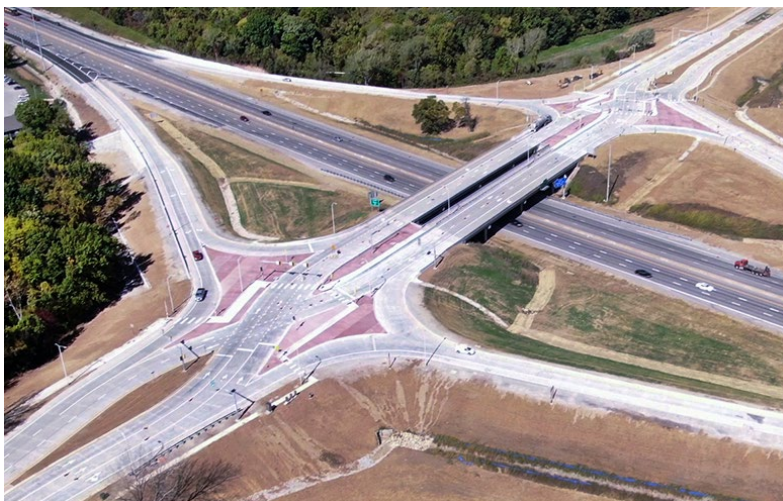
Turner Diagonal project in Kansas City.
