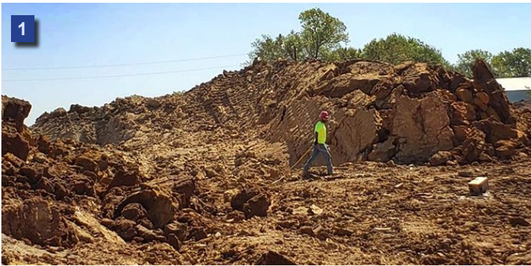
1. Blaster-in-charge checks the area before giving the all clear. 2. Equipment moves material from the post blast excavated area. 3. Workers measure tomorrow's blast grid. Photos by Kate Craft, District One
