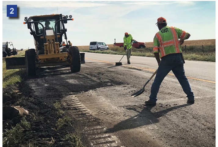
The Jetmore and Ness City Subarea crews patch a large pothole on K-156 west of Jetmore recently. 1. LeRoy Keith and Michael Parker wait as Shannon Moore places asphalt on the patch. 2. Keith and Moore clean up asphalt as Larry Kjellberg prepares to smooth the asphalt out with the motor grader. 3. Kjellberg works the asphalt using the motor grader while the crews clean up loose asphalt behind the motor grader.
