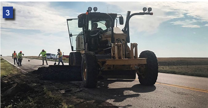
The Jetmore and Ness City Subarea crews patch a large pothole on K-156 west of Jetmore recently. 1. LeRoy Keith and Michael Parker wait as Shannon Moore places asphalt on the patch. 2. Keith and Moore clean up asphalt as Larry Kjellberg prepares to smooth the asphalt out with the motor grader. 3. Kjellberg works the asphalt using the motor grader while the crews clean up loose asphalt behind the motor grader.
