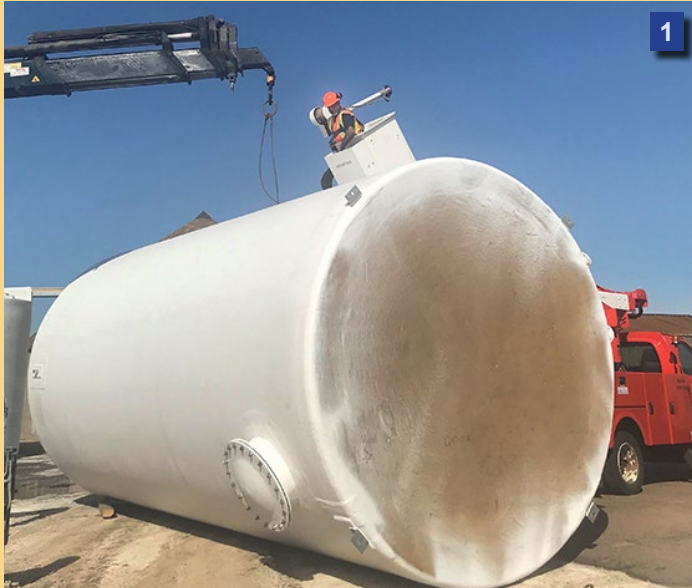
The Garden Subarea received a new 20,000-gallon brine tank on Sept. 24. The new tank will boost the Subarea's brine capacity to 50,000 gallons and allow it to provide brine to other crews as needed this winter.
