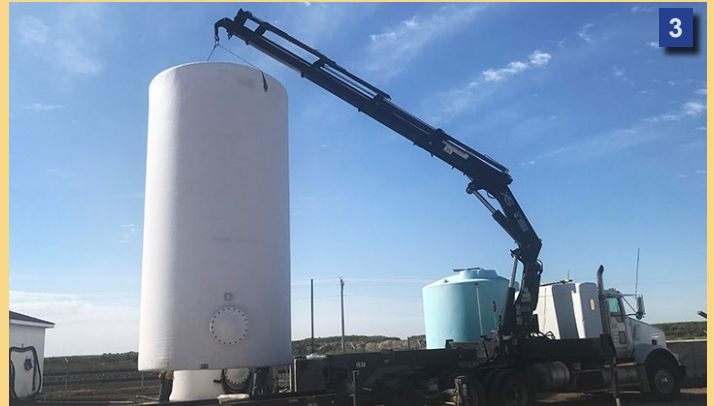
1. Garden City Subarea Supervisor Hector Terrones attaches the crane cables to the tank using the bucket truck. 2. Terrones stands approximately 5,000 gallons tall next to the 20,000-gallon tank. 3. The tank is placed on the concrete deck with the two brine tanks. All photos by Lisa Knoll.
