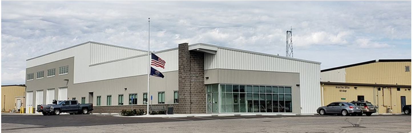
Construction of the new Area Four Gage facility was completed recently. Photos by Kate Craft, District One
