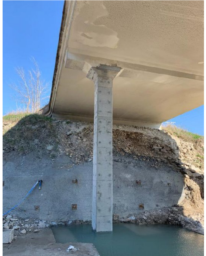
B & B Bridge constructed a new bridge column under K-39 as an emergency repair. Photo provided
