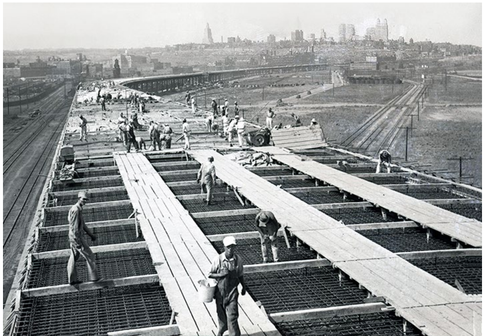
A historical look from a similar view to the photo above of viaduct construction in 1962. Archive photo from Multimedia Services
