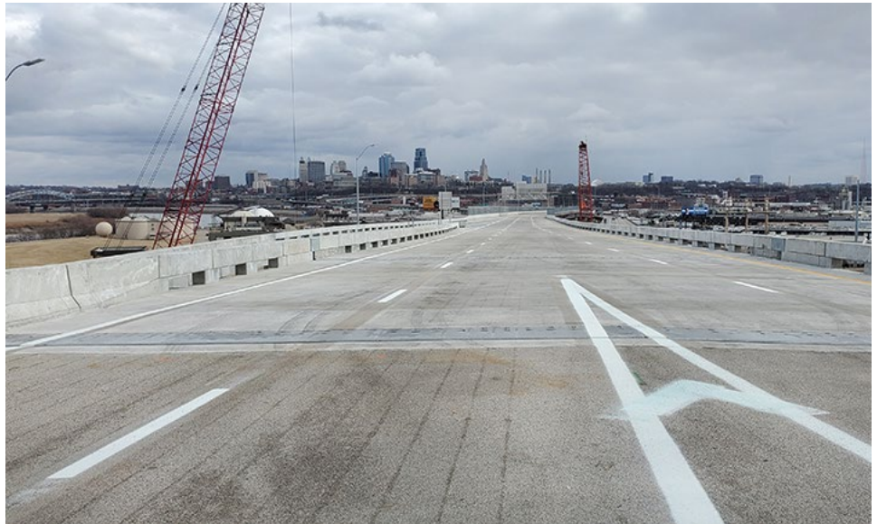
An eastbound view of the new westbound I-70 lanes on the Lewis and Clark Viaduct that opened on Jan. 23. Photo by Joel Smith, District One
