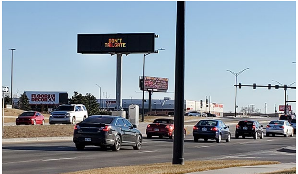
This DMS sign on southbound Webb Road in Wichita helps alert drivers of incidents before they exit onto U.S. 54. Photo by Tracy Crockett, District Five.
