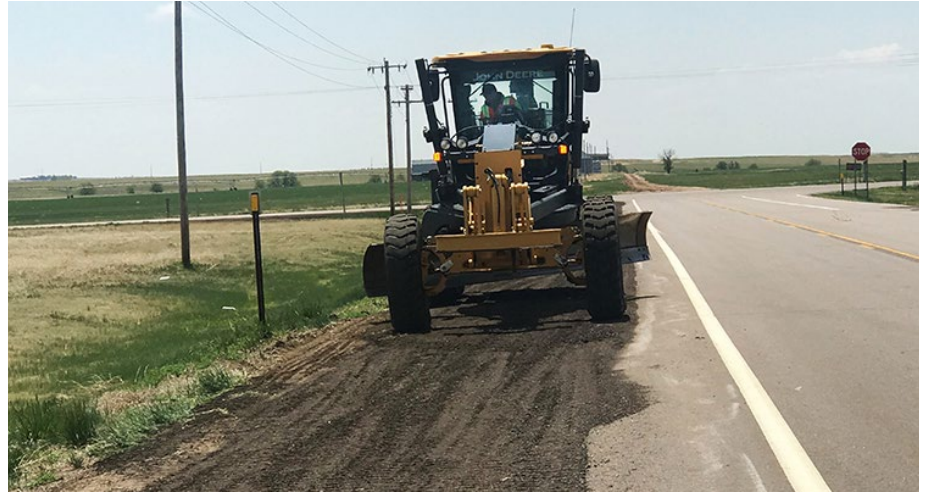
Above, Kent Hall, Equipment Operator at Rolla, fills edge ruts on K-51 in Morton County. Bottom left, Subarea crew members, including Michael Edmondson, Calvin LaMaster and Joseph Ethridge, repair signs on U.S. 56 at Rolla. Photos by Lisa Knoll, District Six
