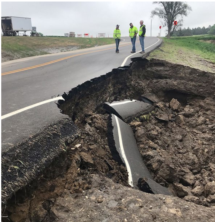
In the photos above and below, floodwaters completely submerged the shoo-fly detour on the K-18 bridge project near Luray, washing away a portion of the roadbed and pavement.
