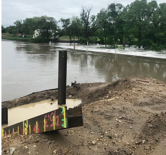
In the photos above and below, floodwaters completely submerged the shoo-fly detour on the K-18 bridge project near Luray, washing away a portion of the roadbed and pavement.
