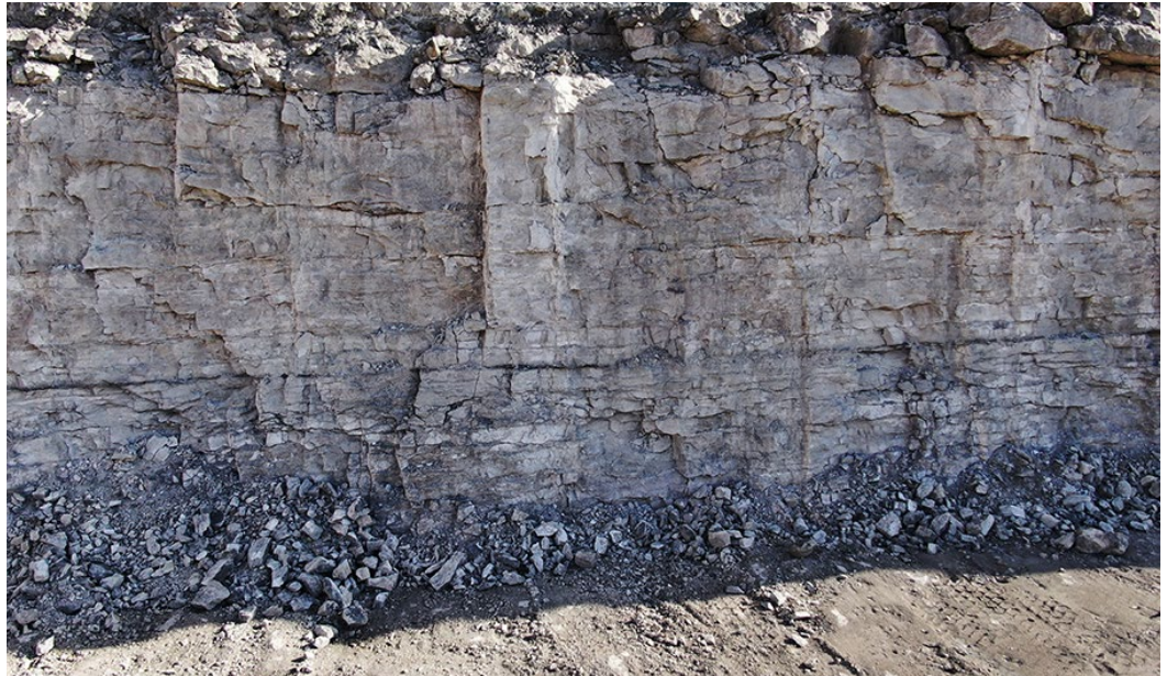
Getting images of the ledge face in a quarry using a drone was accomplished on Dec. 8. Photos by Kyle Halverson, Headquarters
