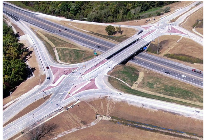
The new Turner Diagonal Interchange project was honored by the American Public Works Association. Photo by KDOT Multimedia
