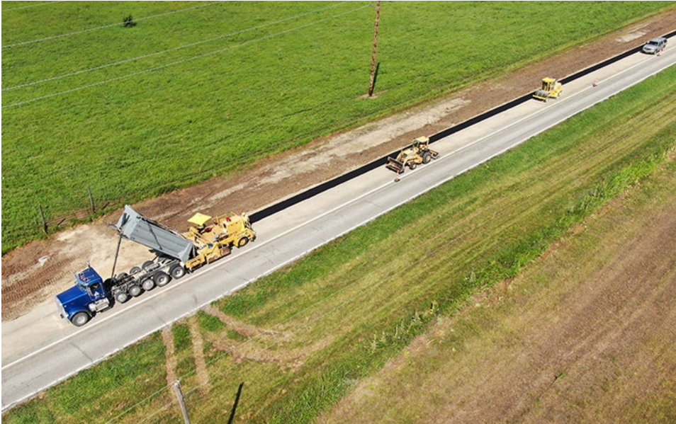
Above and below, drone photos show work on KDOT's project that will add three-foot shoulders on 13 miles of K-99 from Sedan north to the Chautauqua-Elk county line. Two of KDOT's licensed drone operators, Warren Ebberts and Rowden Glaser, took these aerial views to show the progress. Cornejo & Sons of Wichita is the primary contractor on the $8 million project. Work started in May and will continue through the spring of 2022. Jeff Sims' road squad and Brad Rognlie's bridge squad designed the project.
