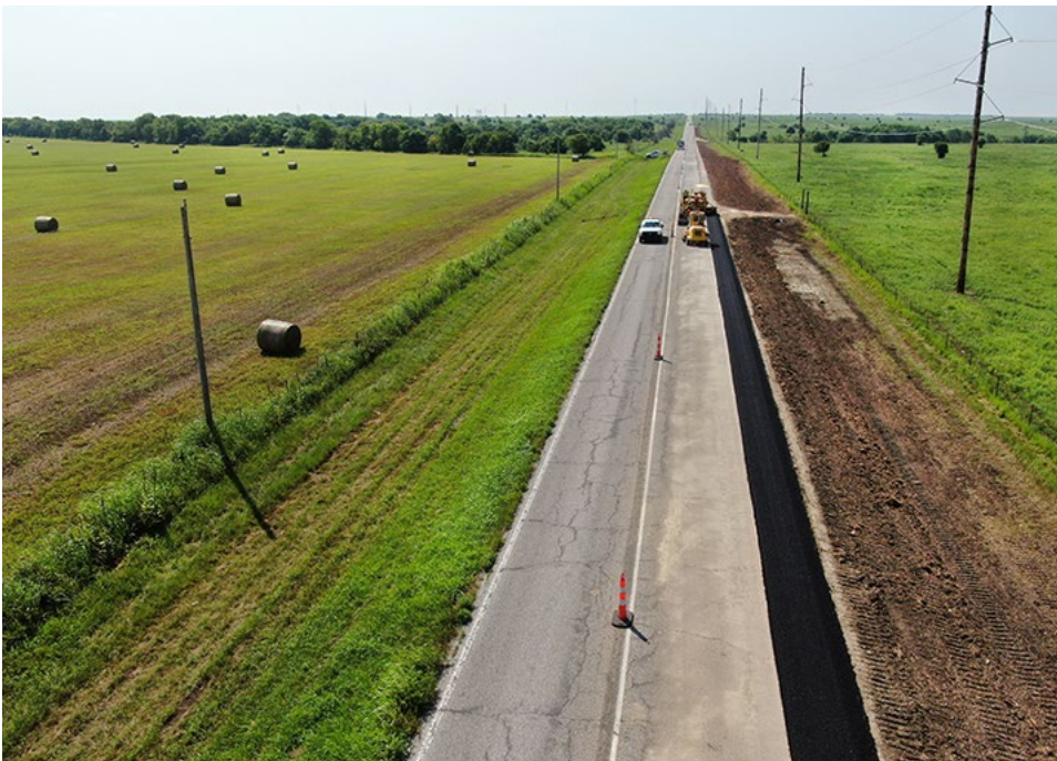
Above and below, drone photos show work on KDOT's project that will add three-foot shoulders on 13 miles of K-99 from Sedan north to the Chautauqua-Elk county line. Two of KDOT's licensed drone operators, Warren Ebberts and Rowden Glaser, took these aerial views to show the progress. Cornejo & Sons of Wichita is the primary contractor on the $8 million project. Work started in May and will continue through the spring of 2022. Jeff Sims' road squad and Brad Rognlie's bridge squad designed the project.
