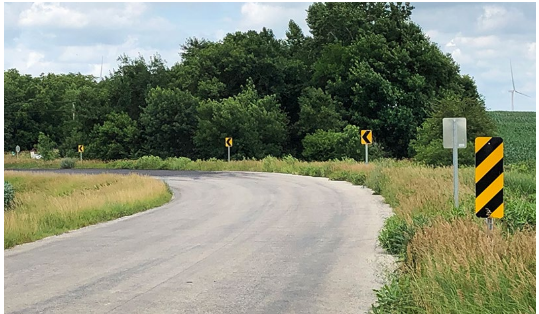
Signing was improved along this Rural Major Collector road in Nemaha County to reduce roadway departures. This project was developed through the Bureau of Local Projects. Photo by Dawn Hueske, Headquarters
