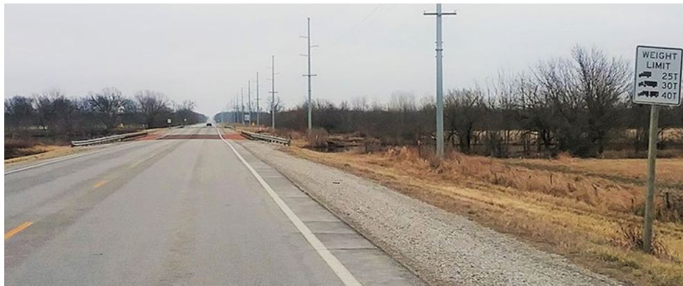
Each of the six existing U.S. 166 bridges is posted for weight limits, and is considered ‘scour critical.’ KDOT awarded Bridges Inc., of Newton the $14.8 million construction contract. Photo by Priscilla Petersen, District Four
