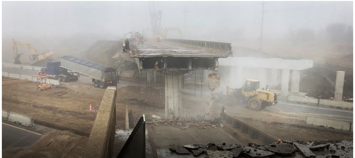
Above, demolition required full closure of I-35 for less than 24 hours. Below, girders are set over piers. Photos by Ali Al Inizi, District One
