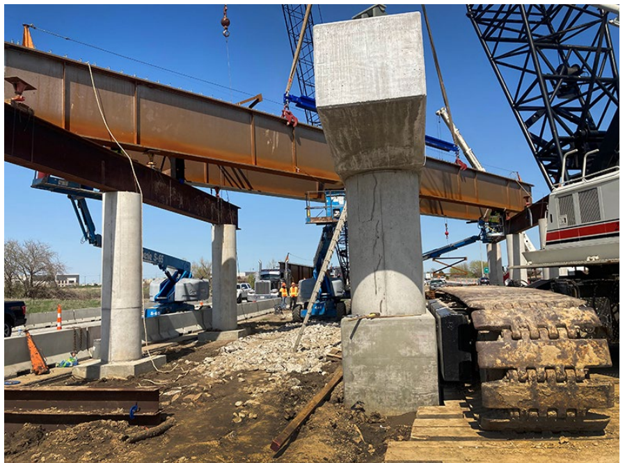
Above, demolition required full closure of I-35 for less than 24 hours. Below, girders are set over piers. Photos by Ali Al Inizi, District One
