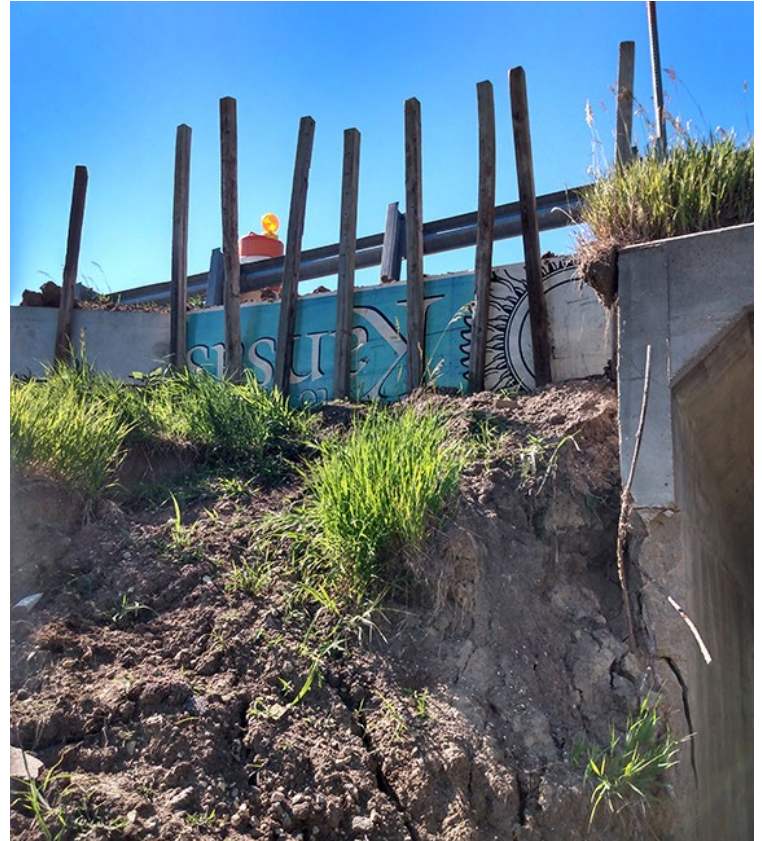
An old "Welcome to Kansas" sign shows resources can come from anywhere as crews used it to temporarily shore up the eroding embankment until the emergency repair job could be completed.
