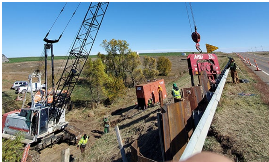
An old "Welcome to Kansas" sign shows resources can come from anywhere as crews used it to temporarily shore up the eroding embankment until the emergency repair job could be completed.
