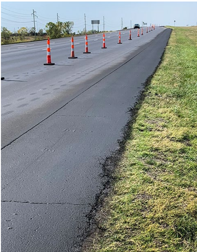
High Density Mineral Bond, or HA5, has been applied to existing shoulders on K-254 near El Dorado as seen in the photos on this page. Photos by Nick Squires, District Five
