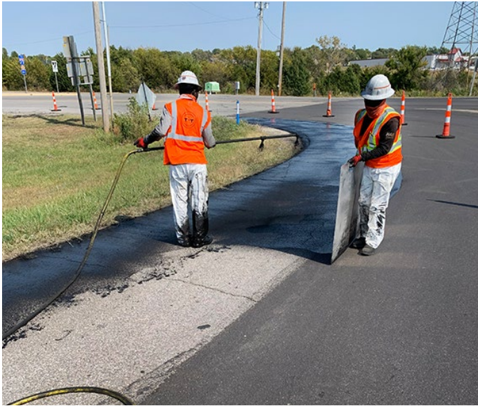
High Density Mineral Bond, or HA5, has been applied to existing shoulders on K-254 near El Dorado as seen in the photos on this page. Photos by Nick Squires, District Five
