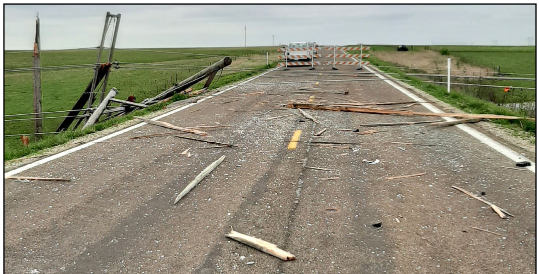
Top photo: This picture provided by the KHP shows the scene with power lines down along I-70 near mile marker 315. Middle and bottom photos: Along K-177, power lines were also down over a pond and debris was strewn along the road. Photos by Kevin Jirak and Randy Kunc, District Two
