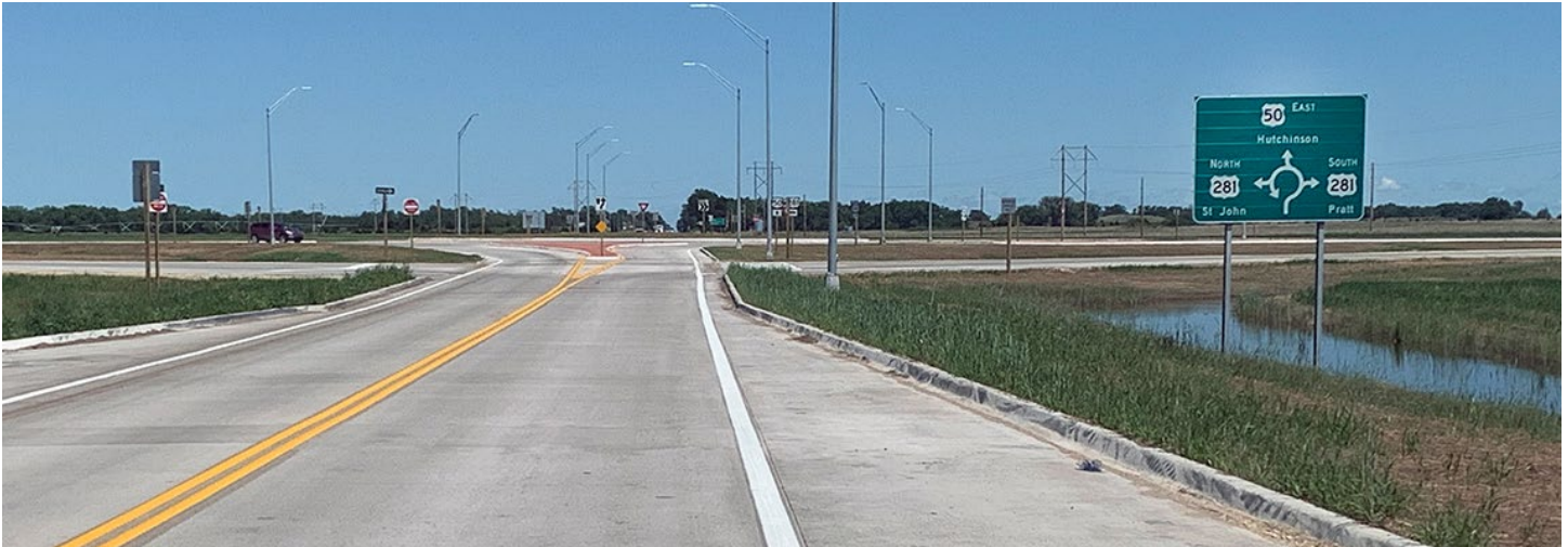
View of the new roundabout at U.S. 50 and U.S. 281, south of St. John. Photo by Doug Coates, District Five
