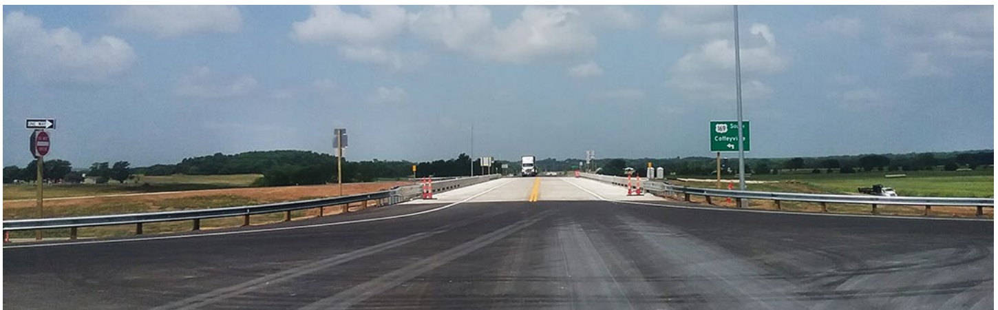
A semi approaches the U.S. 160 bridge over U.S. 169.
