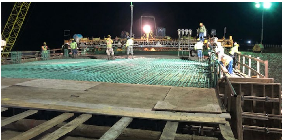
In the photos above and below, crews worked overnight on June 11 to pour concrete for the new span bridge in Gove County carrying westbound I-70 over County Road 62. The multi-year project is in its final construction season with work shifting into the westbound lanes. In addition to constructing the new bridge, the project scope includes replacing the pavement on a 9-mile stretch of the interstate starting one mile west of the K-23 spur near Grainfield and ending four miles east of K-211. The pavement at the westbound rest area near Grainfield will also be replaced. Work on the $38.1 million project is expected to be completed by the end of November. Debbie Tanking's road squad and Brad Rognlie's bridge squad designed the project. Photos by Todd Anderson, District Three
