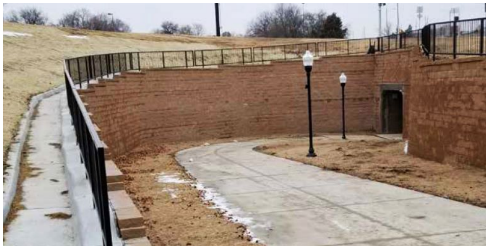
The $6.9 million bicycle and pedestrian underpass project in Lawrence. Photo provided by the City of Lawrence
