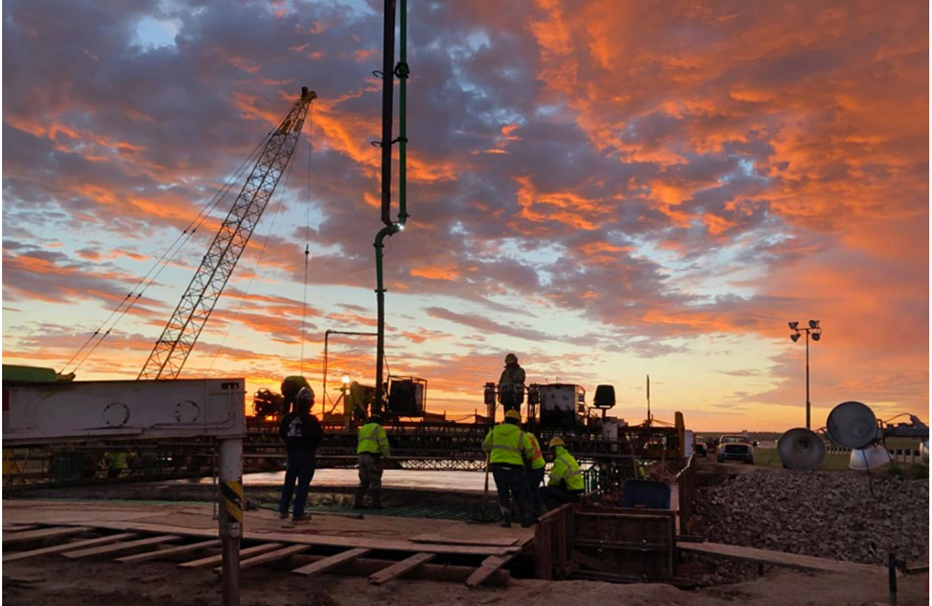
In the photos above and below, crews worked overnight on June 11 to pour concrete for the new span bridge in Gove County carrying westbound I-70 over County Road 62. The multi-year project is in its final construction season with work shifting into the westbound lanes. In addition to constructing the new bridge, the project scope includes replacing the pavement on a 9-mile stretch of the interstate starting one mile west of the K-23 spur near Grainfield and ending four miles east of K-211. The pavement at the westbound rest area near Grainfield will also be replaced. Work on the $38.1 million project is expected to be completed by the end of November. Debbie Tanking's road squad and Brad Rognlie's bridge squad designed the project. Photos by Todd Anderson, District Three
