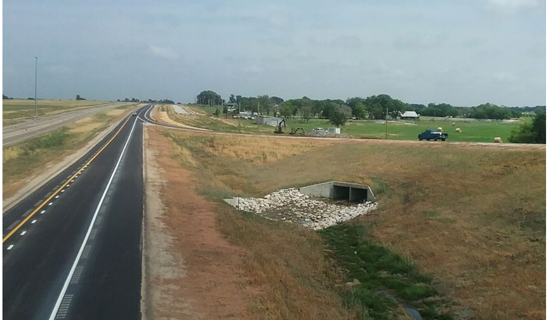
A truck is about to enter the northbound lanes of U.S. 169 from one of the ramps now open at the interchange. Photos by Priscilla Petersen, District Four
