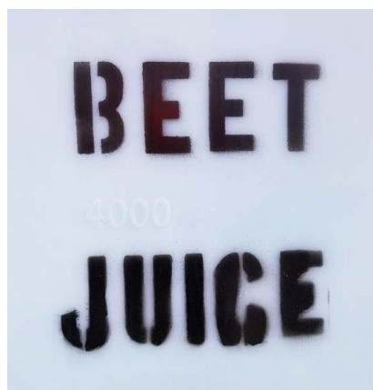
A "beet juice"-labeled storage tank in Wichita. The juice is a byproduct of sugar beet processing.
