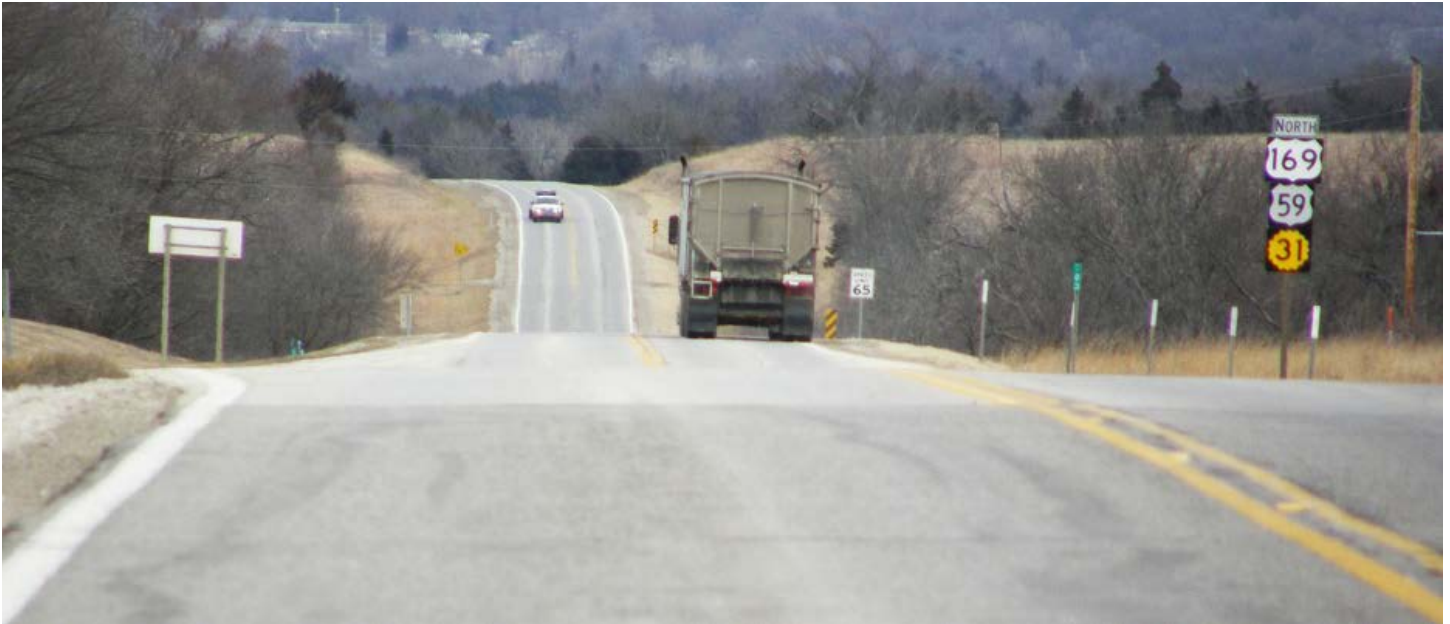
In March, KDOT plans to start construction on a previously delayed T-WORKS project to reconstruct 7½ miles of U.S. 169 from Welda north to Garnett. The south section, from Welda to the U.S. 59 junction, will be fully reconstructed with 12-foot lanes and 10-foot shoulders. The existing two lanes will be rehabilitated and 10-foot shoulders will be added to the section north of U.S. 59, pictured. Bettis Asphalt & Construction Company, Inc., of Topeka is primary contractor on the $21 million project. KDOT is holding a groundbreaking for this project on Feb. 21 at Welda. Greg Gonzales' road squad and Shawn Schwensen's bridge squad designed the project. Photo by Priscilla Petersen, District Four
