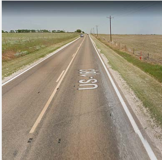
Photos show a section of U.S. 160/183 south of Coldwater before and after 2-foot shoulders were added. Now, KDOT plans to add shoulders on U.S. 183 north of Coldwater, in Comanche County, and continuing into Kiowa County.
