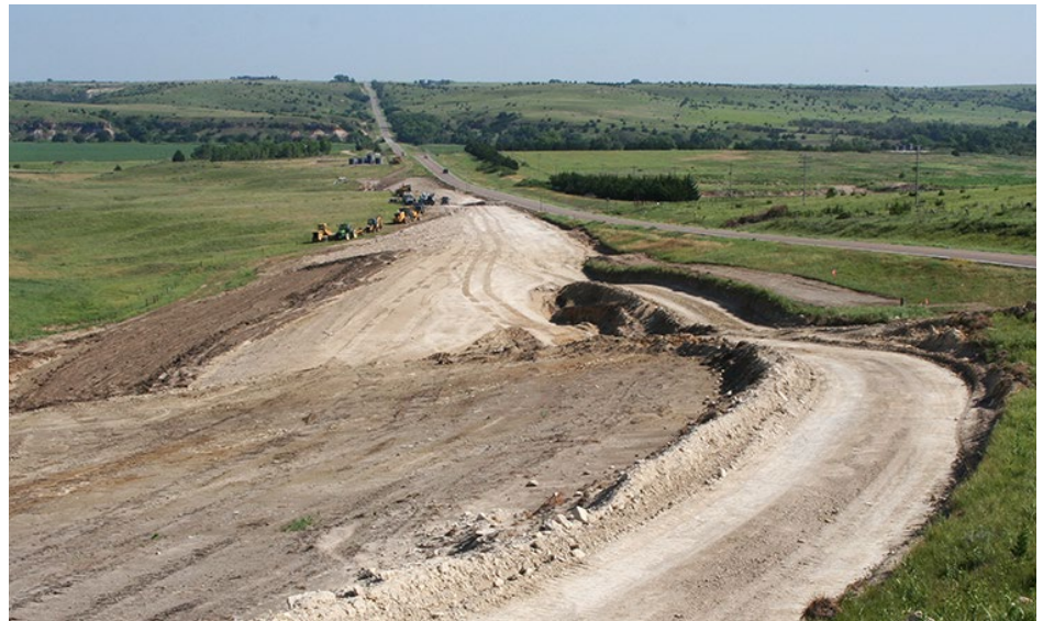
Above: Grading work takes place on U.S. 281. At left: Crews work on cutting in to nearly 50 feet of rock to form the backslope in the west ditch on the northern end of the realignment piece. Note the difference in color between the rock at the top and bottom of the formation. Regional Geologist Neil Croxton explained that both are the same kind of rock, except the light colored has been exposed to the elements while the dark portion has been buried in the earth. Photos by Neil Croxton
