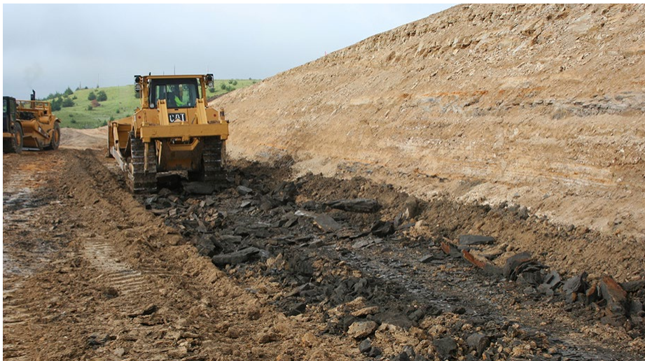
Above: Grading work takes place on U.S. 281. At left: Crews work on cutting in to nearly 50 feet of rock to form the backslope in the west ditch on the northern end of the realignment piece. Note the difference in color between the rock at the top and bottom of the formation. Regional Geologist Neil Croxton explained that both are the same kind of rock, except the light colored has been exposed to the elements while the dark portion has been buried in the earth. Photos by Neil Croxton
