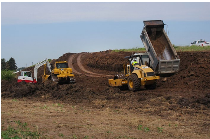
Grading work and building the bridge approaches have begun, as seen in the photos above and at right. Photos by Ashley Perez, District Two
