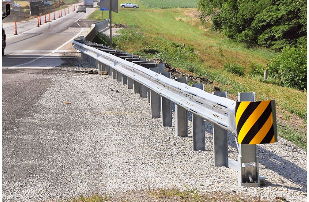
Recently installed guardrail on U.S. 59 near Garnett. Photo by Multimedia Support
