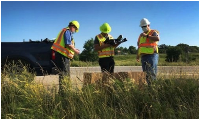
KC Scout members coordinate installation for the day.
