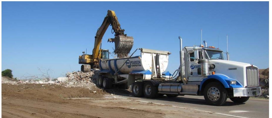
To protect the road surface from the heavy equipment, a dirt cushion was placed over the concrete lanes. Photos by Tom Hein
