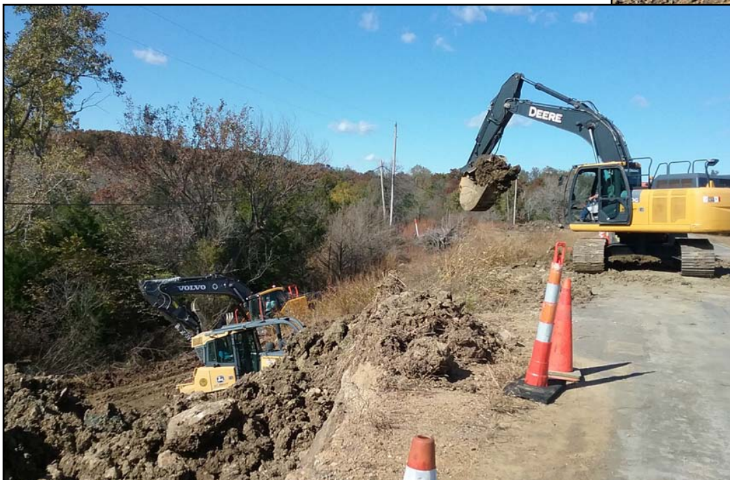
Above, Geologist Denny Martin inspects a fabric mat placed on the ground at the slide. Rock and concrete will be placed on top of the mat, which will act as a filter. At left, Crews work to repair a major slide along K-105 north of Cross Timbers State Park. Photos by Denton Decker and Priscilla Petersen, District Four
