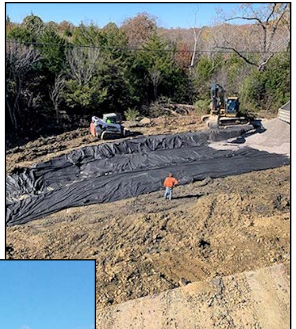
Above, Geologist Denny Martin inspects a fabric mat placed on the ground at the slide. Rock and concrete will be placed on top of the mat, which will act as a filter. At left, Crews work to repair a major slide along K-105 north of Cross Timbers State Park. Photos by Denton Decker and Priscilla Petersen, District Four
