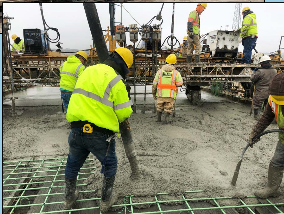
Above, concrete was placed on the new westbound Kellogg bridge crossing Greenwich in Wichita. This project will ultimately provide new direct access to the KTA and the Turnpike is managing the project. You can learn more about the East Kellogg project at www.e54ict.com . At right, concrete was placed on the 30th Street South bridge crossing I-35/KTA near the Southern Terminal.
