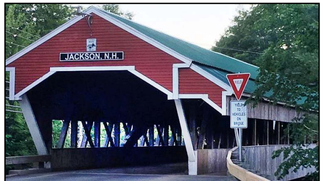
Bridge photo: New Hampshire DOT
