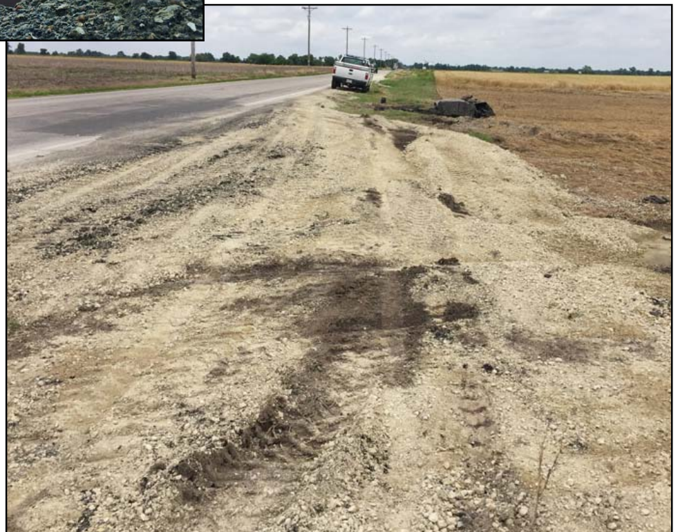
Above, is the monster hole KDOT workers tackled south of Lyons along K-14/K-96. Flooding gouged out the hole next to the pavement. The hole was 20 feet wide, 30 feet long, up to 6 feet deep. Photos by Randy Miller, District Five.
