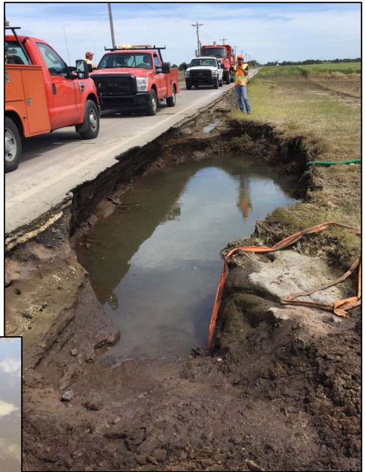
Above, is the monster hole KDOT workers tackled south of Lyons along K-14/K-96. Flooding gouged out the hole next to the pavement. The hole was 20 feet wide, 30 feet long, up to 6 feet deep. Photos by Randy Miller, District Five.
