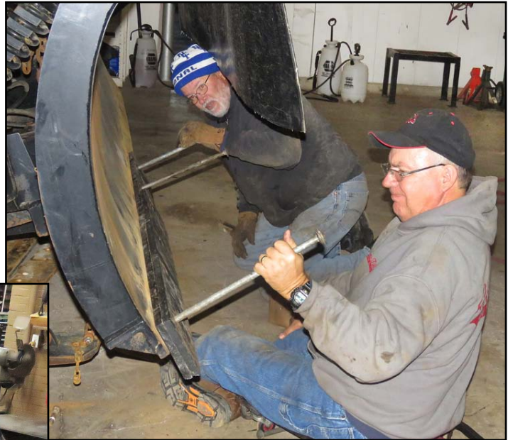
Above, Equipment Operators Charles Seabolt and Tim Harris replace blades on the snow plow in Ulysses while below, Equipment Operator Edwin Pineda checks the spray pattern on the brine truck.
