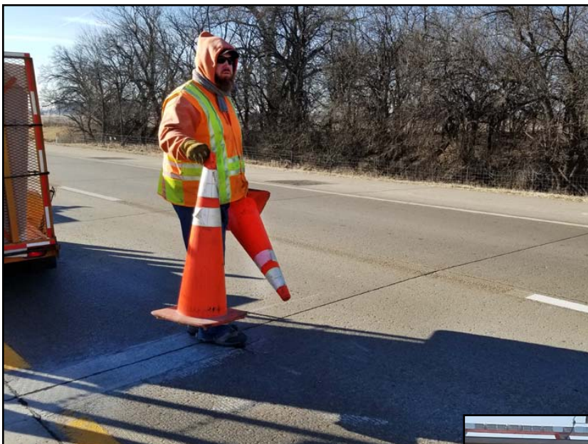
Above: Equipment Operator Rocky Lindgren places cones to move traffic over (seen at top right) in preparation for guardrail repair work.
