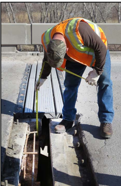
Above, Landon Baier from the District Bridge Crew removes debris from beneath the expansion joint. Below, Justin Mead measures for the concrete form.
