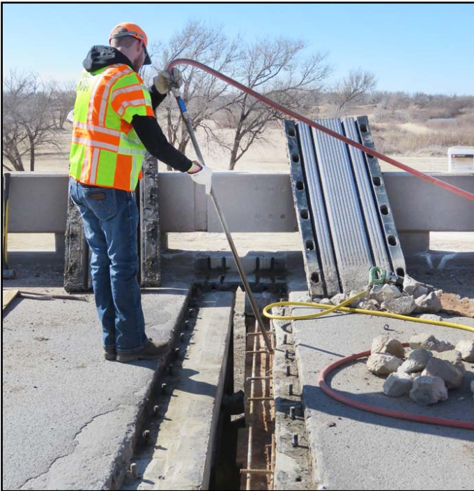
Above, Landon Baier from the District Bridge Crew removes debris from beneath the expansion joint. Below, Justin Mead measures for the concrete form.
