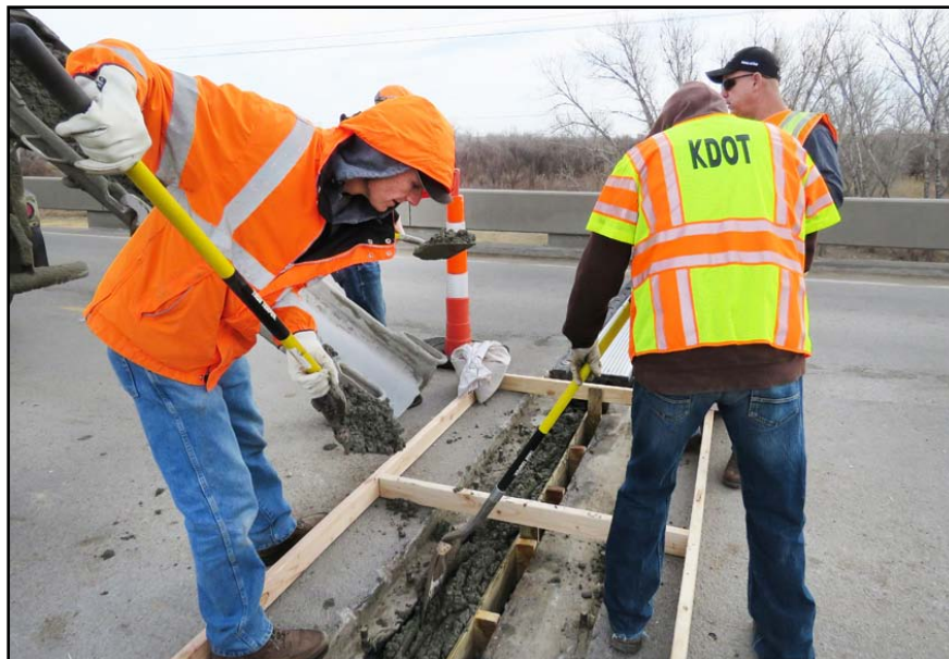
The bridge crew places concrete to support the expansion joint.
