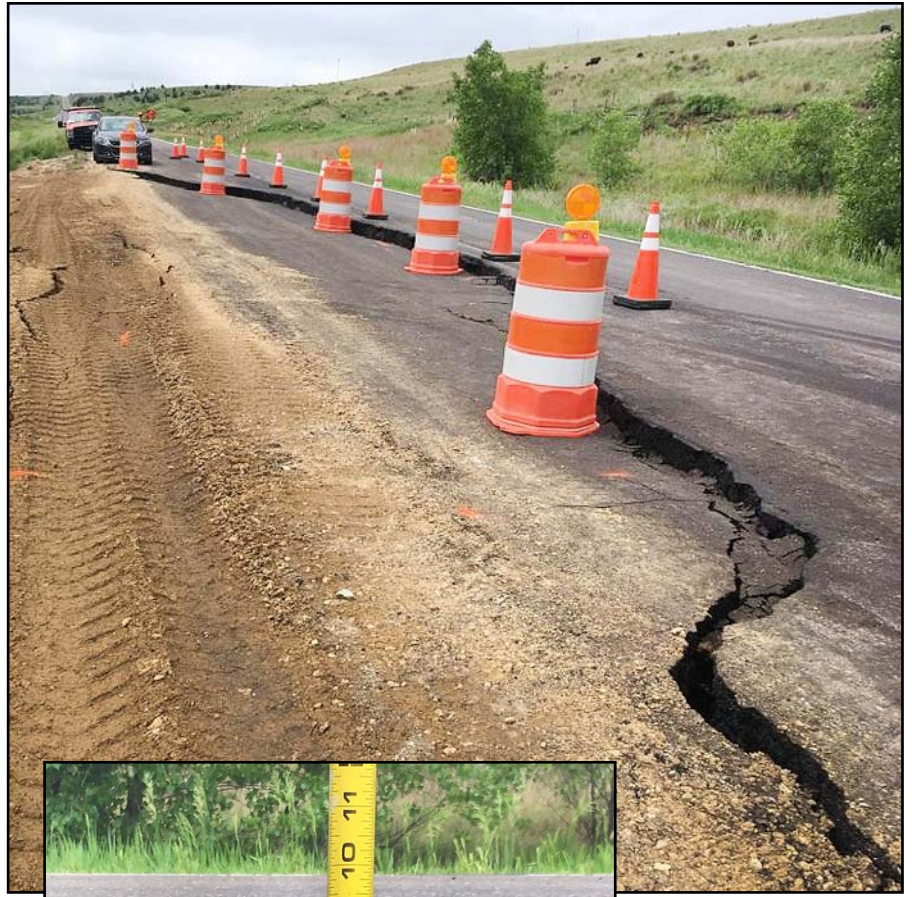
Above: A flagging operation had to begin on May 28 as the slide on U.S. 281 got worse. Far left: A picture of the highway on May 13 shows the highway slide starting. Left: This photo taken May 29 shows the eight-inch drop in the pavement.
