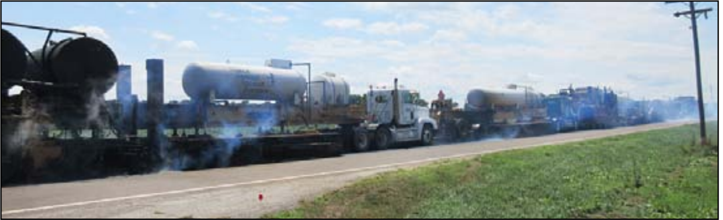
A variety of work is underway in District Two - above, a hot-in-place recycle takes place on K-18 in Ottawa County; below left, the District paint crew stripes K-4 just south of Dwight; and below right, the Clay Center Subarea patches overlays on K-15 north of Clay Center.
