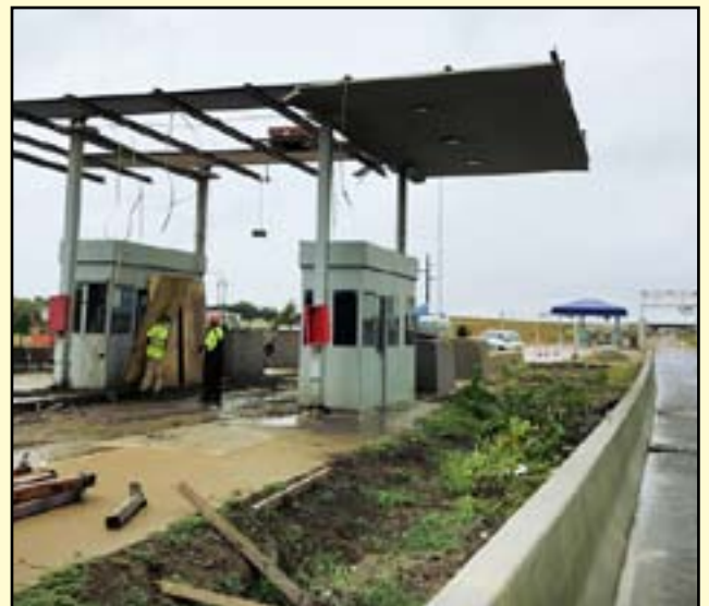
Construction on the new KTA East Topeka plaza is coming along. Crews prepared the roadway to set a high-mast light pole and worked on tearing down the old toll booths last week.
