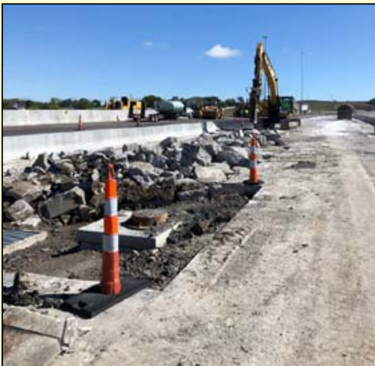
Construction on the new KTA East Topeka plaza is coming along. Crews prepared the roadway to set a high-mast light pole and worked on tearing down the old toll booths last week.
