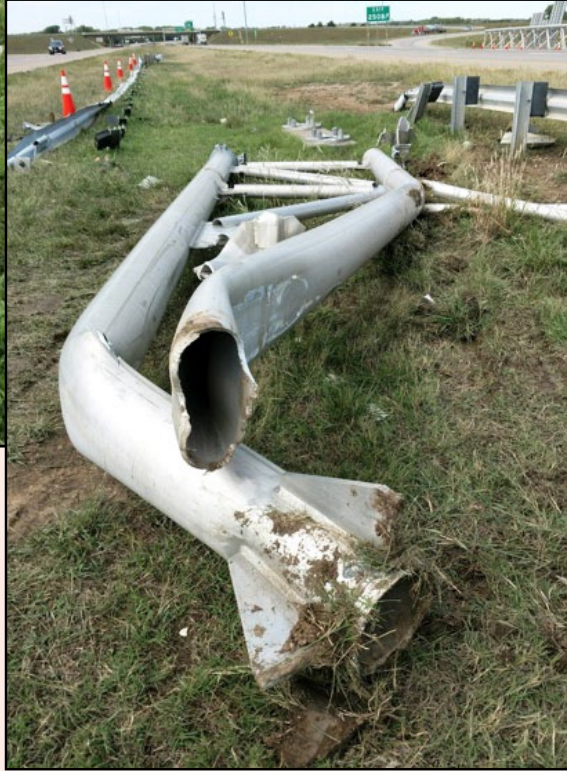
Above and right, the support column for the overhead sign on I-70 near the I-135 junction was destroyed in a crash on Sept. 28. Below, work takes place to replace the columns and install the sign.
