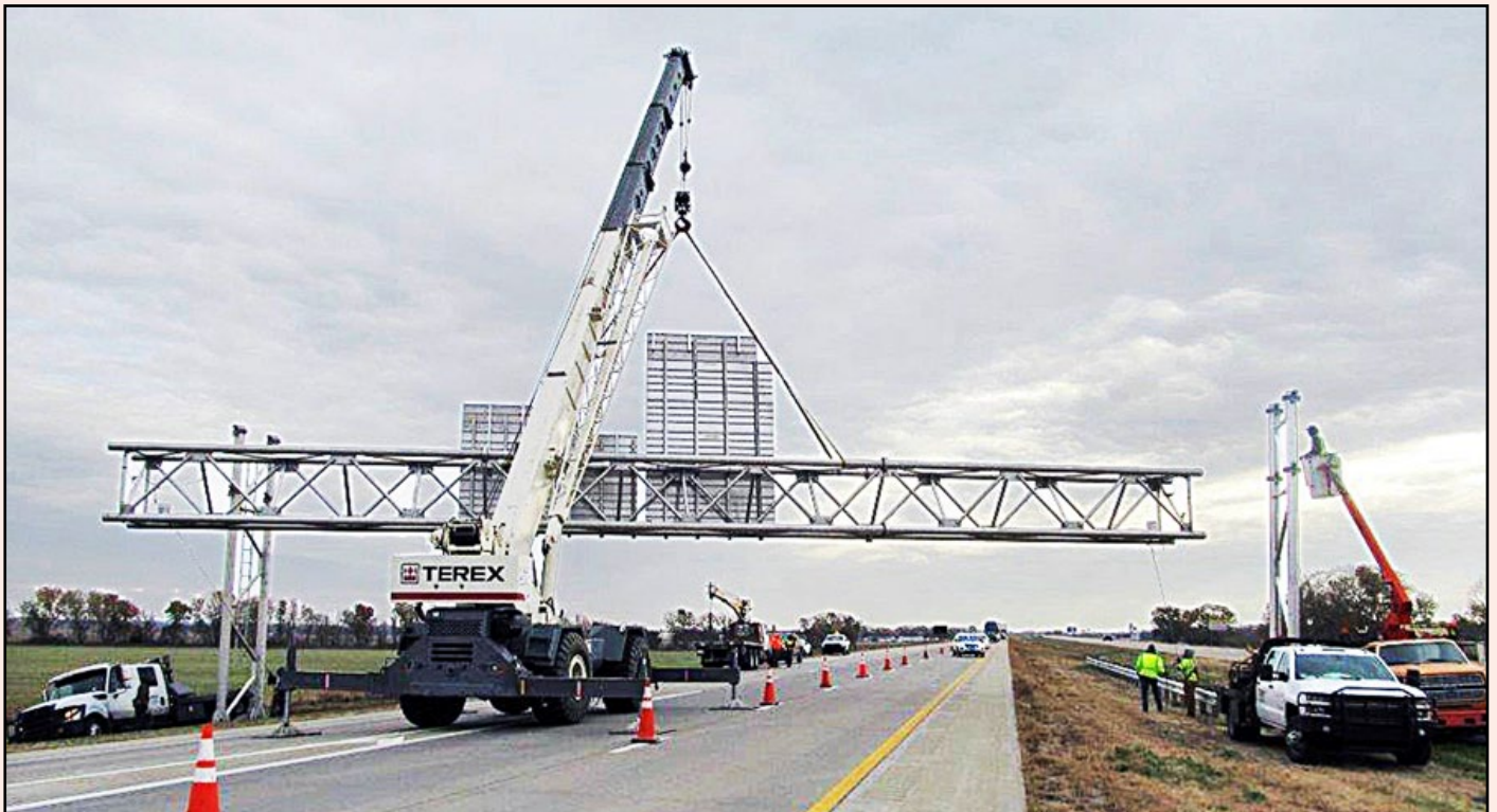
Above and right, the support column for the overhead sign on I-70 near the I-135 junction was destroyed in a crash on Sept. 28. Below, work takes place to replace the columns and install the sign.
